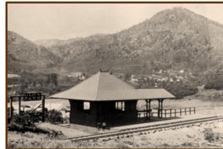
Above left: Glen Park D&RG railroad station, ca 1888
